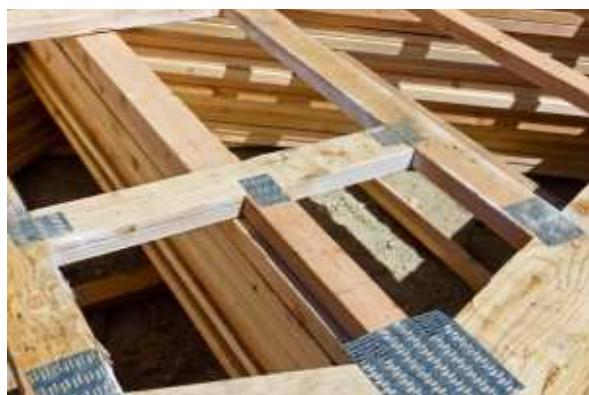
2. **MITERED BUTT JOINT:** The mitered butt joint is very similar to the standard butt joint, in that it typically joints two boards at their ends, or one board at an end meeting the side of another board. The difference is in how those ends meet. In a standard butt joint, the end or ends are left square so they meet at a 90 degree angle. In a mitered butt joint, the end or ends are mitered to a 45 degree angle. This allows two boards to turn a corner
