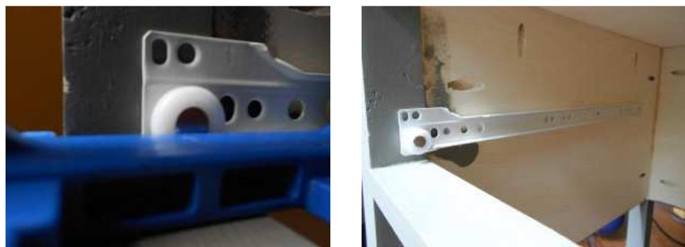
8. Attach the drawer-side hardware to the bottom of the drawer and make any necessary adjustments.
