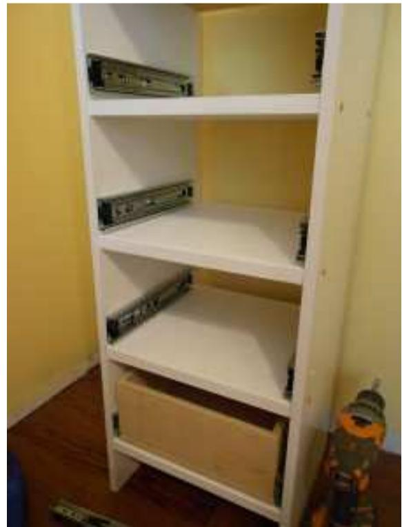
5. Remove the jig and attach the drawer hardware to the drawer. The hardware can also be removed if it makes it easier to attach the hardware.
