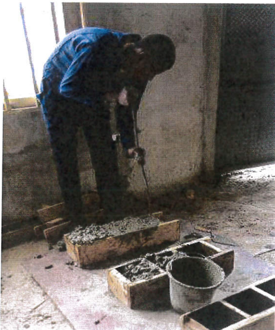
Plate 3.9 Tamping of concrete
