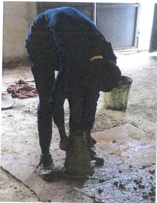
Plate 3.15 Lifting of slump cone
