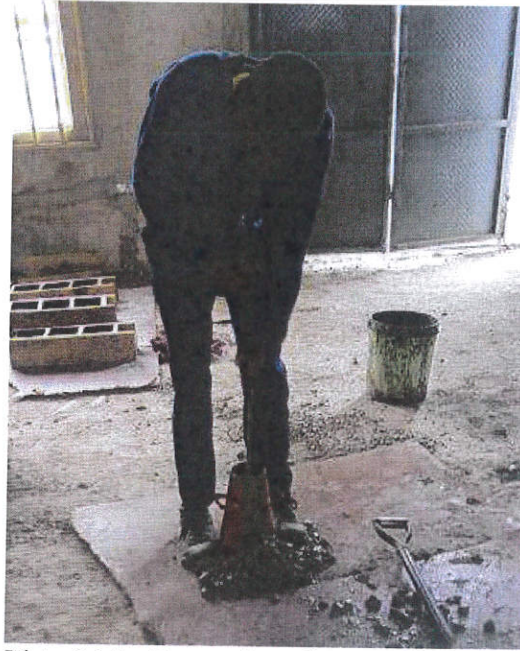
Plate 3.14 Tampering of concrete
