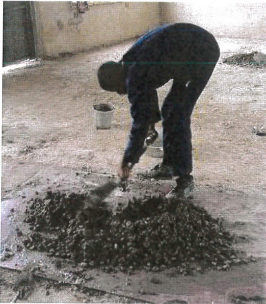
Plate 3.8 Mixing of Concrete
