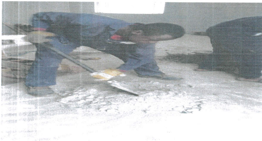
Plate 3.13 Mixing of Concrete
