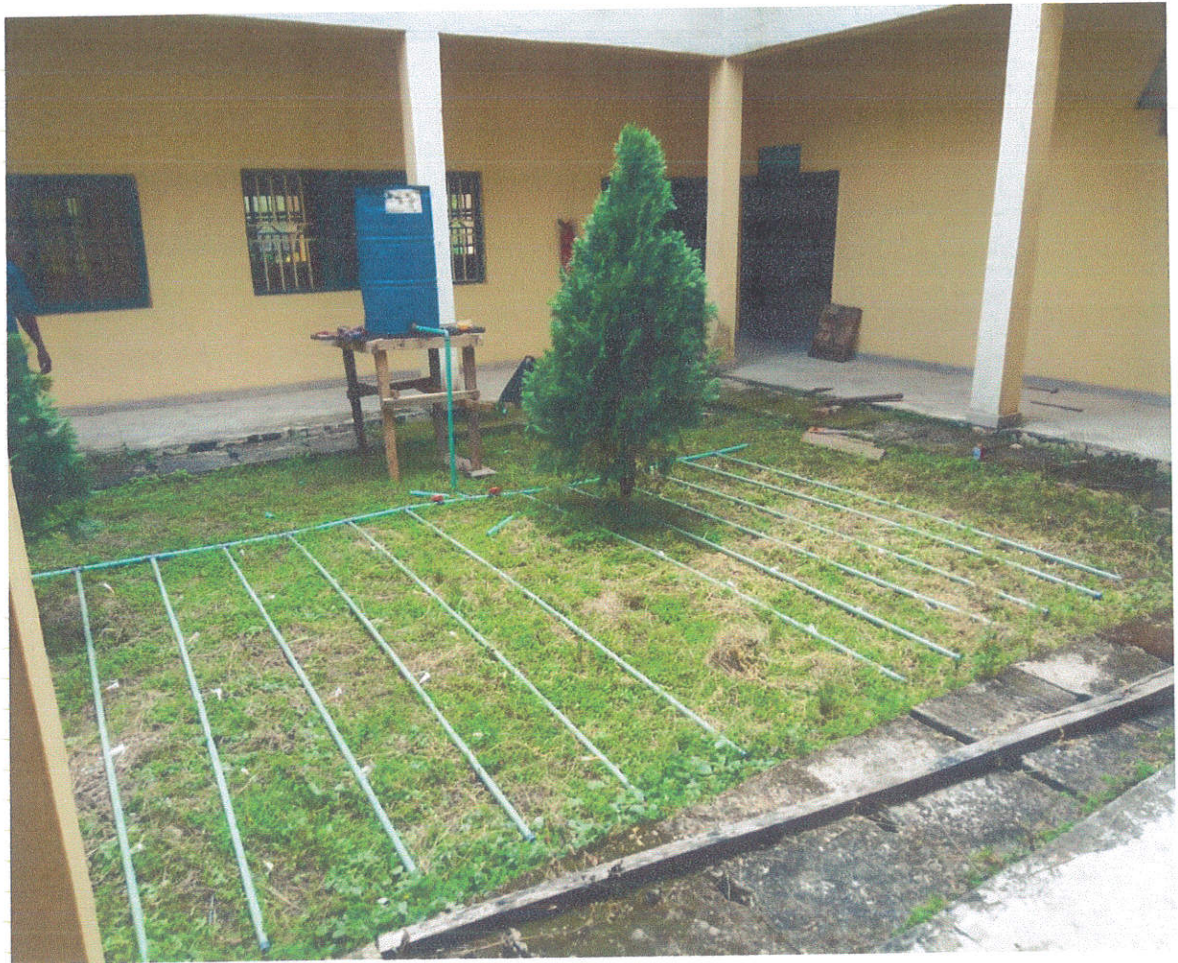
Figure 3.7: Field Layout Gravity Drip Irrigation System
