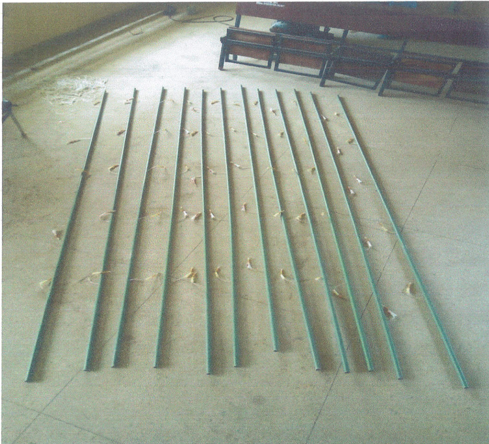
Figure 3.4 Lateral lines fixed with Hospital Drip Flow
